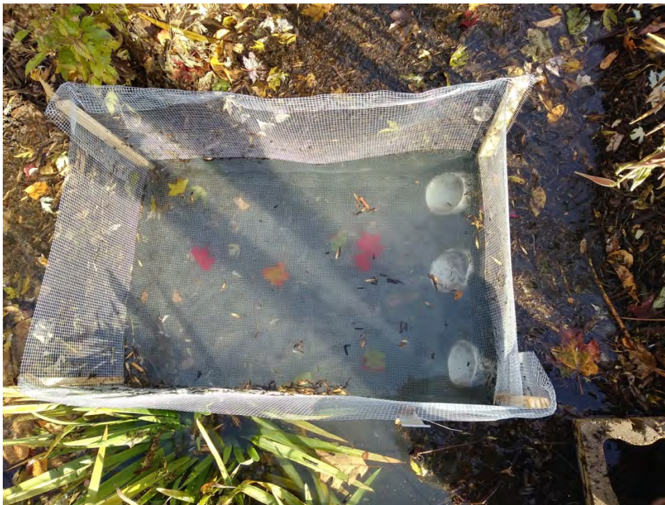
Figure 23. Gross solids containment area at Bloomington field site. Flow from the shallow sump box enters the bioretention basin through the three pipes at right.
