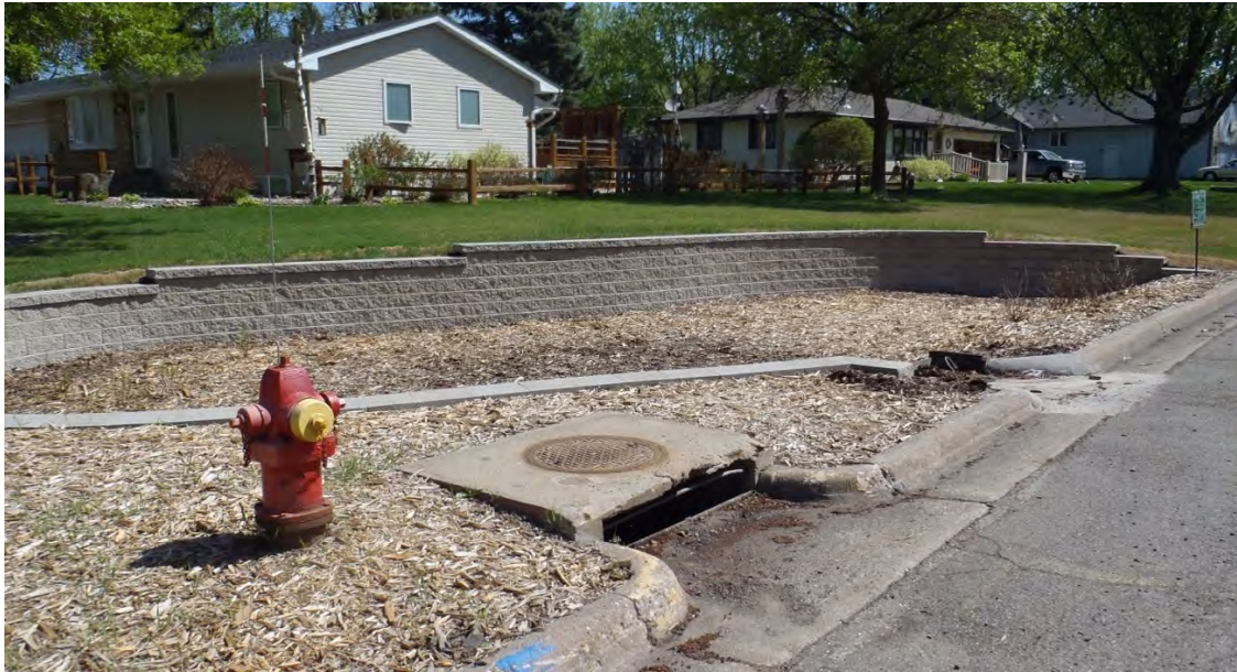
Figure 1. Photo of the Anoka site in May 2018, prior to testing. Gutter flow along 38 th Lane is from right to left in the photo, encountering the basin inlet before the large catch basin nearest the fire hydrant.
