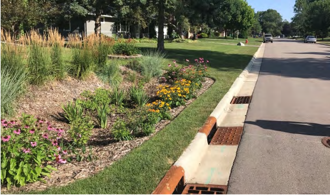
Figure 5. Queen Avenue rain garden in Bloomington, looking north. The inlet to the pretreatment device is through the furthest curb grate. The gutter low point is between the middle and bottom catch basins.
