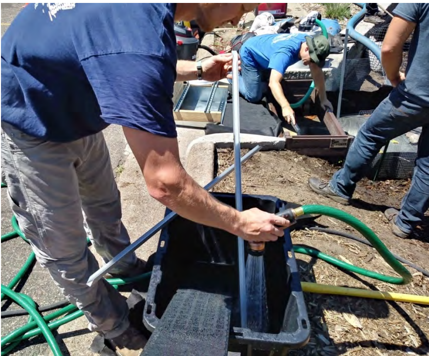
Figure 36. Rinsing the partially disassembled Rain Guardian Bunker screen wall in a bin (foreground) and vacuuming captured sediment from the bunker (background).
