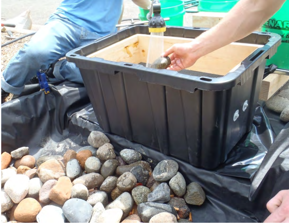
Figure 44. Rinsing rocks from the rock lined inlet.
