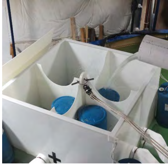
Figure 4 Effluent Sampling Location Situated above the Filter Box
