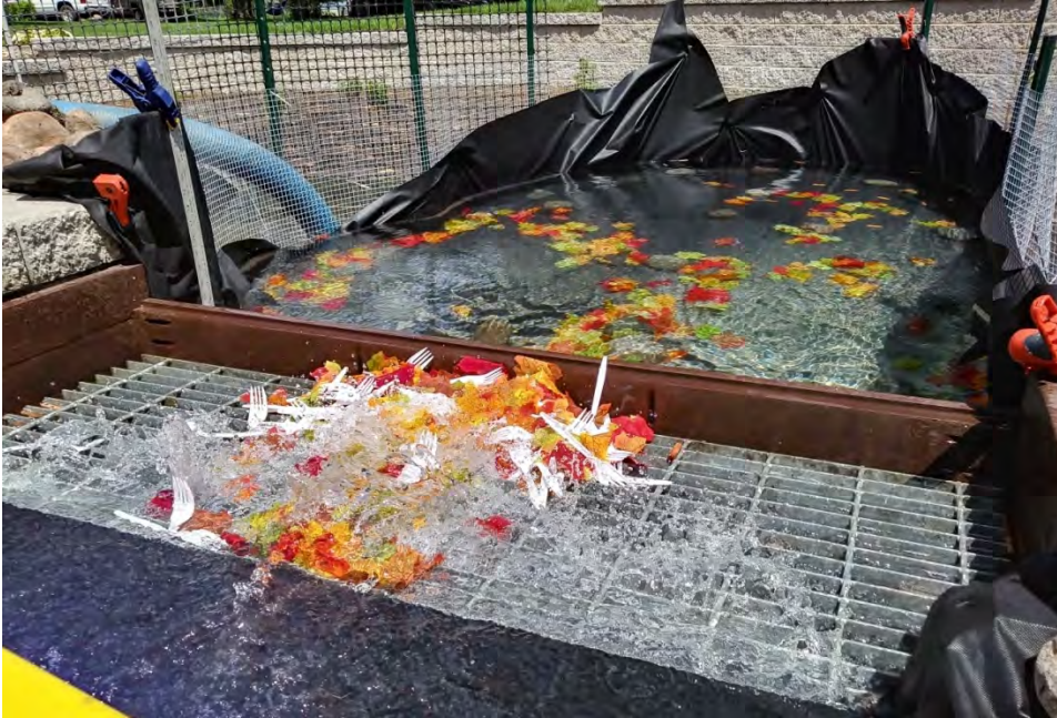
Figure 35. Rain Guardian Bunker at 0.5cfs test flow (RGB-050-A)
