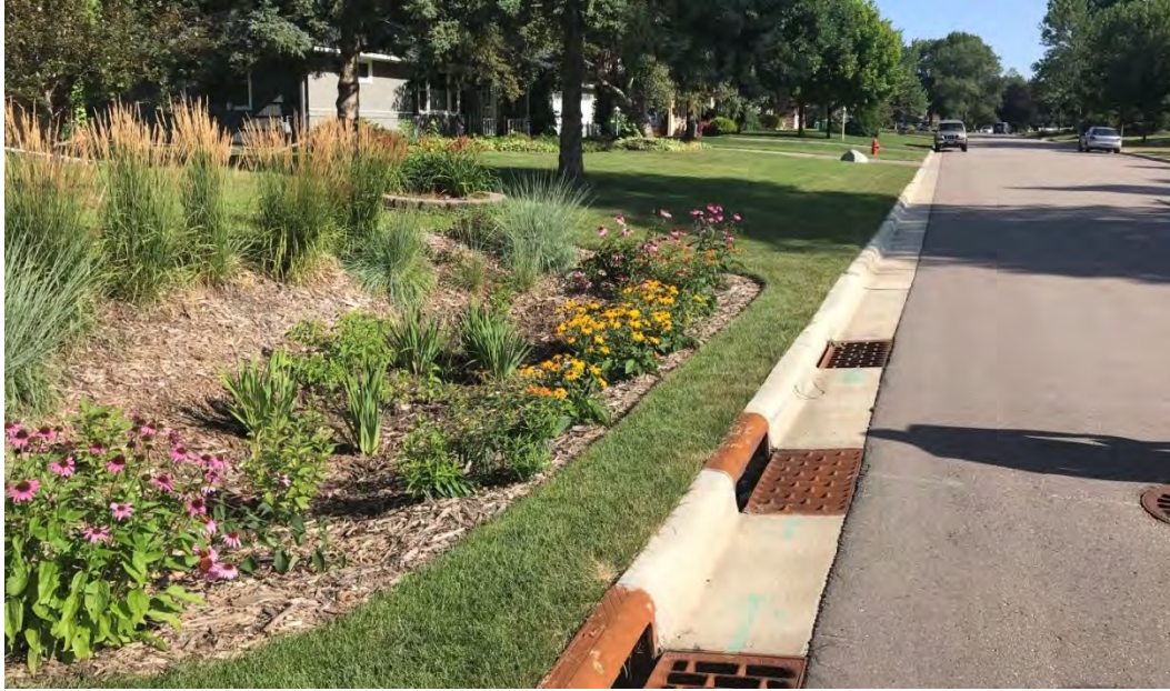
Figure 5. Queen Avenue rain garden in Bloomington, looking north. The inlet to the pretreatment device is through the furthest curb grate. The gutter low point is between the middle and bottom catch basins.
