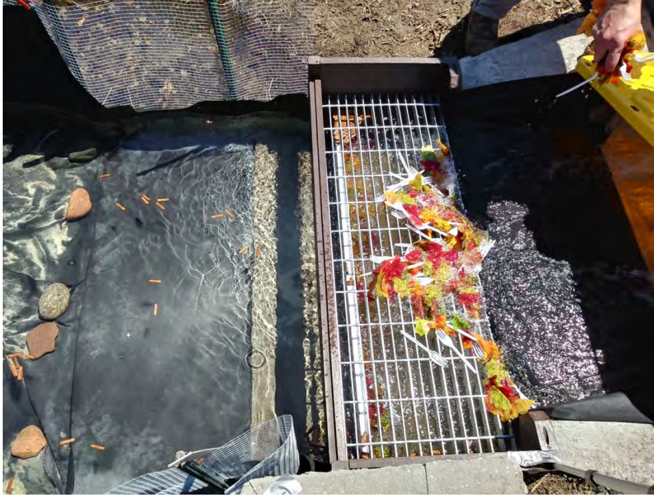
Figure 8. Overhead view of Rain Guardian Bunker (RGB) at 0.25 cfs during gross solids addition (RGB-025-B). Entrance from the curb cut comes into the RGB from the right of the picture; flow through the screen wall exiting the RGB in the center of the picture towards the left.
