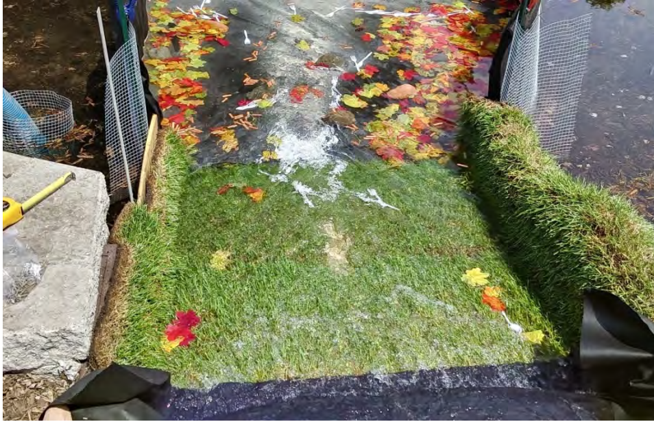
Figure 7. Flow on grass lined inlet at 0.25 cfs (GLI-025-B). Curb cut entrance along bottom of the picture, exit into the bioretention practice at the top.
