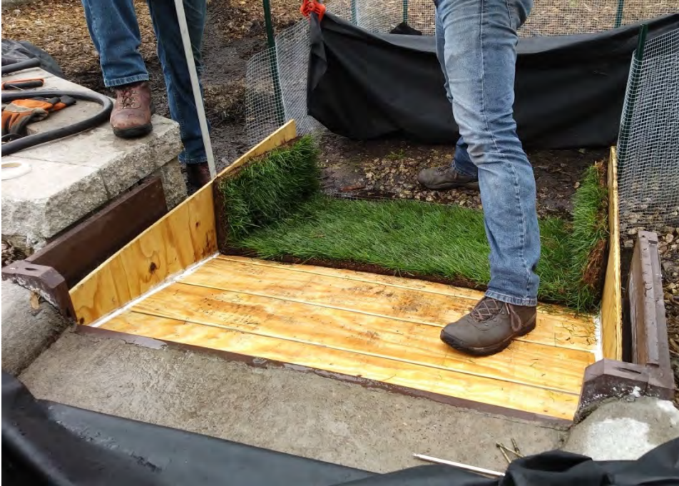
Figure 31. Preparing the grass lined inlet with fresh sod.
