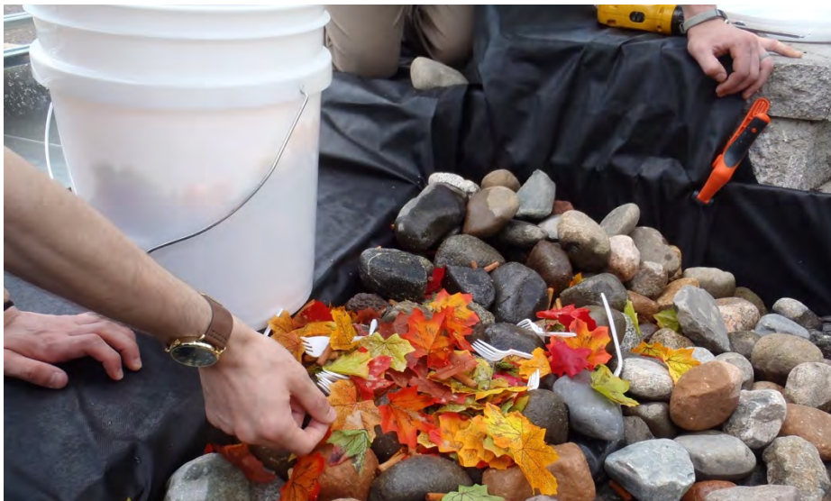
Figure 43. Removal of gross solids from the rock lined inlet.
