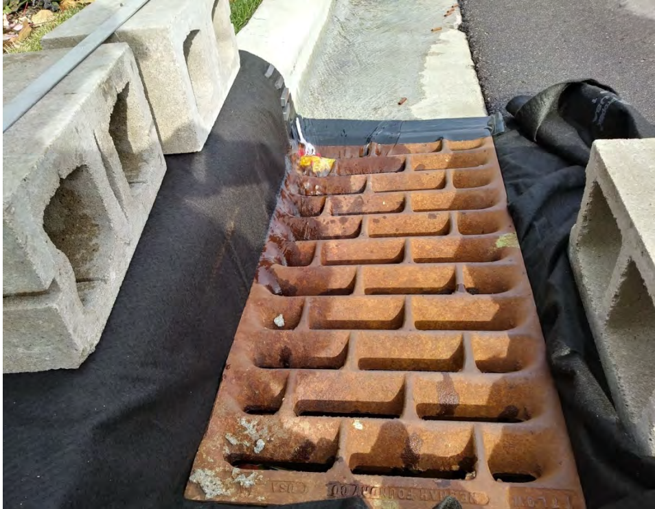
Figure 48. For the bypass tests of the Bloomington pretreatment practice, the downstream catchbasin was lined with a geotextile basket to capture sediment and gross solids bypassing and/or washing out of the pretreatment practice.
