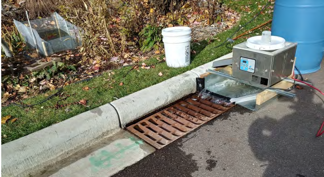
Figure 21. Bloomington field site during pre-wetting flow. Flow enters the shallow sump through the curb grate and emerges into the fenced area of the rain garden through pipes, shown in a subsequent photo.
