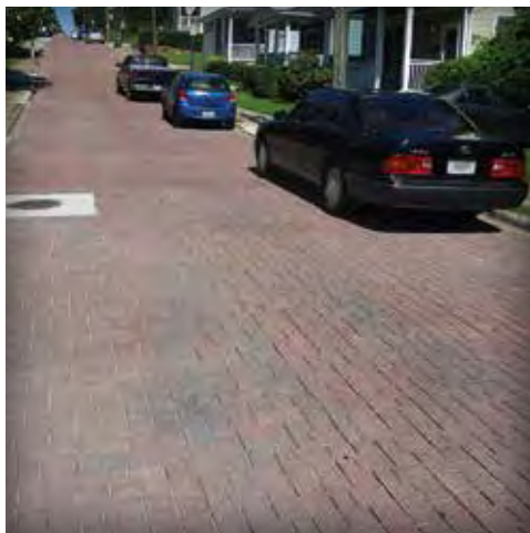
Figure 1. PICP is seeing increased use in municipal streets to reduce stormwater runoff, local flooding, storm pipe upsizing, and combined sewer overflows. These streets are in Atlanta, GA.
