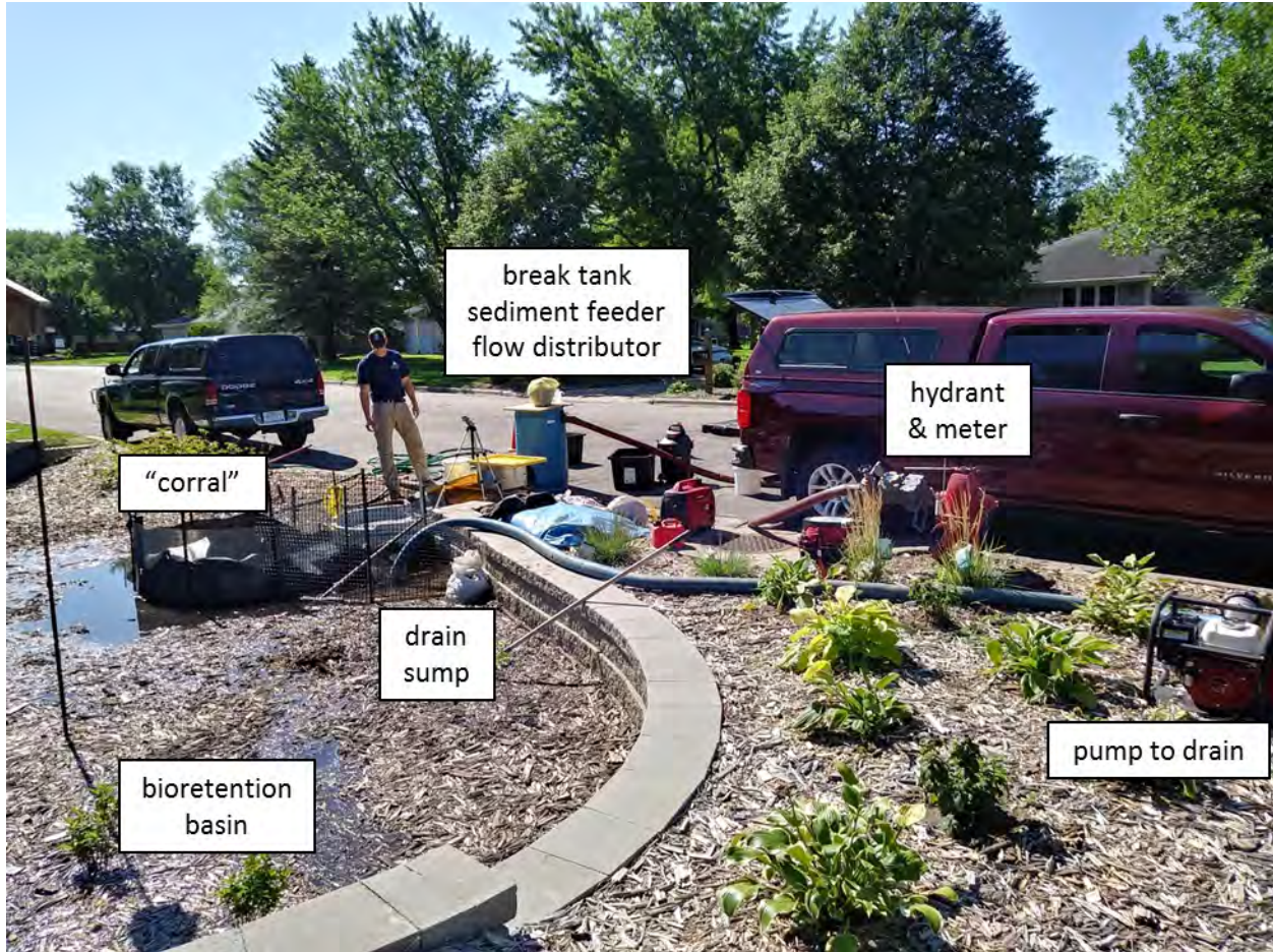
Figure 20. Field equipment used at Anoka field site.
