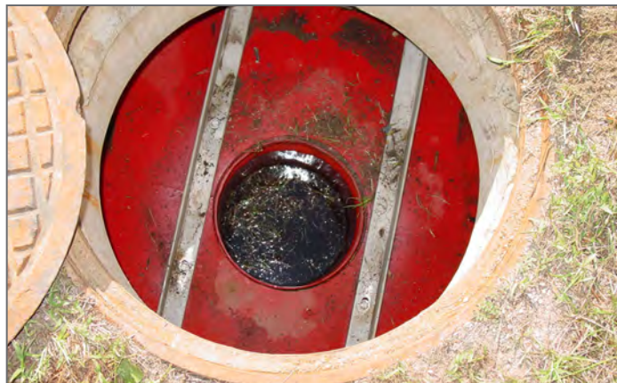
Fig.7 View over center shaft into sediment storage zone.
