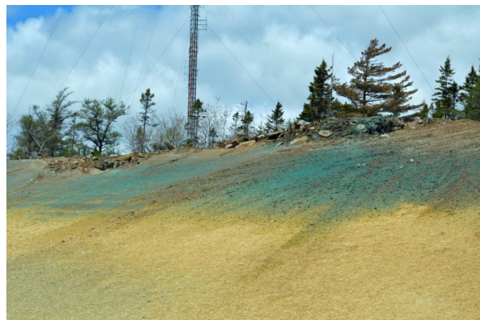
Straw and hydroseed applied to a slope.
