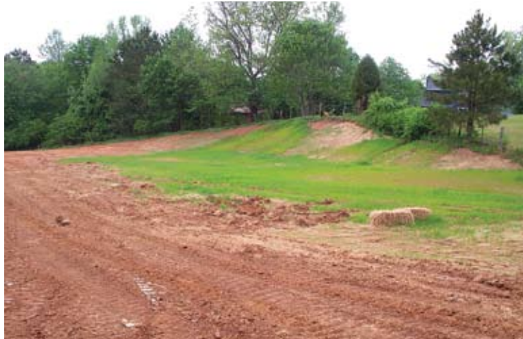
Designate haul roads and material storage areas on large sites, and seed or mulch the rest to minimize the amount of bare areas exposed to the weather.
