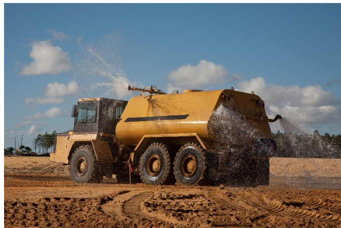
A truck equipped with a spray system can spray water throughout a construction site and prevent dust from being transported off-site.
