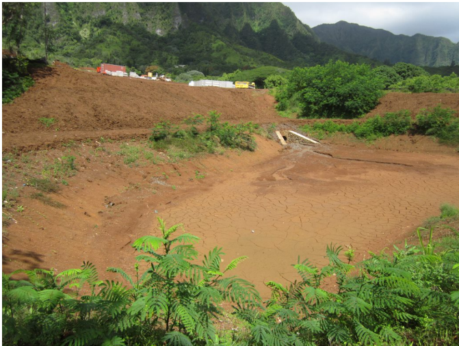
A large sediment basin with partially stabilized embankments.
