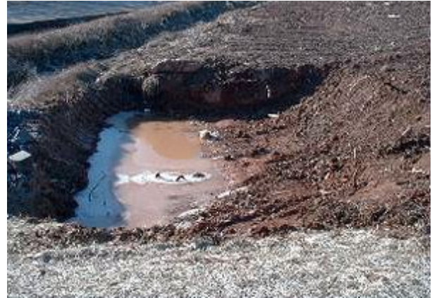
A sediment trap in an unstabilized area with sediment-laden stormwater collected inside.
