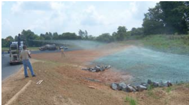
Hydraulically applied seed, mulch, tackifier, and soil amendments (e.g., lime, fertilizer) offer excellent results at a reasonable price on large sites, especially those with long, steep slopes. Follow manufacturer's recommendation regarding materials mixing and application rates.
