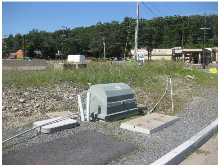
Observed on-site electrical box and exposed conduit.
